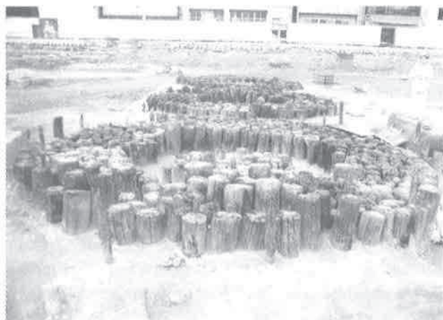
Shiodome site - timber foundation pile clusters, c.1900
