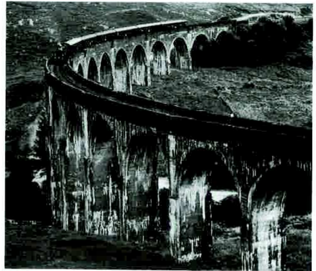
The Panel's 'Special' on Glenfinnan Viaduct 12 July 1997 (courtesy Railtrack)
