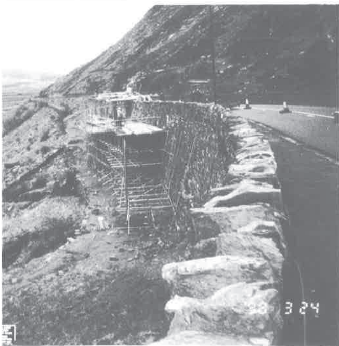
Securing Telford's retaining walls on A5 in Nant Ffrancon Pass
