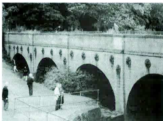
SK 520 598 - King's Mill Viaduct Mansfield & Pinxton Railway (HEW 1775)
