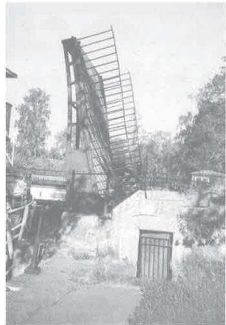
Göta Canal - Forsvite cast iron lifting bridge Author's photograph
