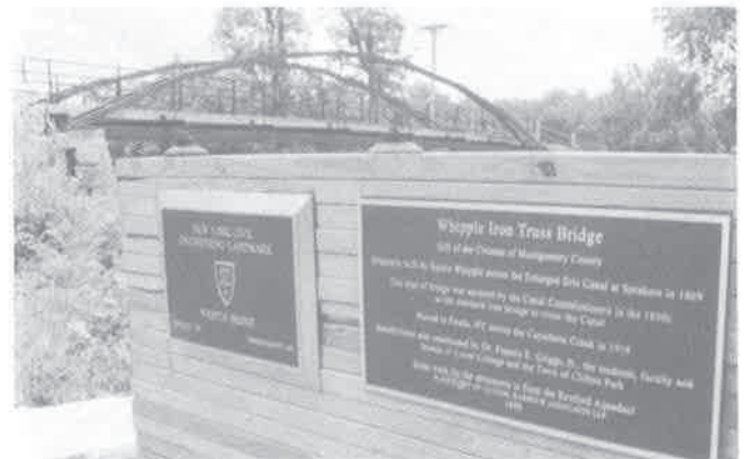
Erie Canal Bridge, Forts Ferry Author's photograph
