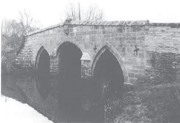
Radcot Bridge, Oxfordshire (HEW 1913)
