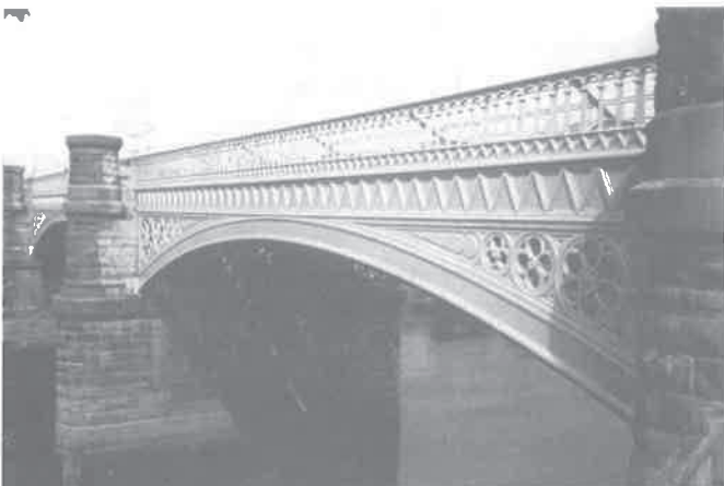
River Lune Bridge, Lancashire (part of HEW 1022)
