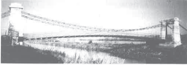
Horkstow Suspension Bridge, North Lincs. (HEW 598)
