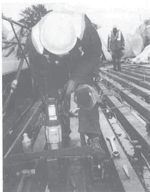
Photograph courtesy of Dorothea Restorations Limited
