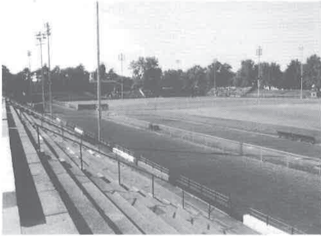
19 th century earth-banked reservoir conserved as Bleecker sports stadium, Albany, N Y State Photograph by Professor Paxton
