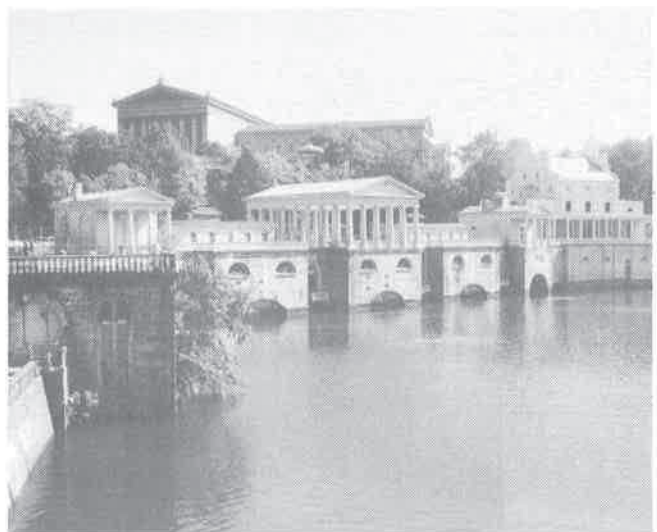
Fairmont Waterworks, Philadelphia (1812-1911) with Museum of Art behind. Note entrance tunnels to waterwheels (c.1821) and engine house (1812-1815) on right © The Author
