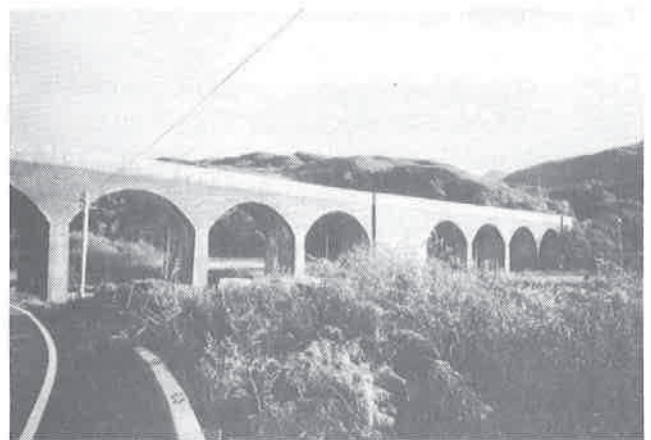
The Loch-nan-Uamh Viaduct (view from west) © The Author
