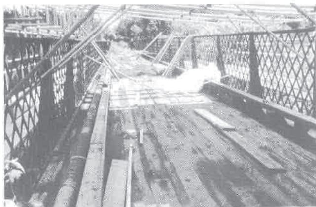
(4) Bilston Glen Viaduct – Deck under construction © Geoff Mather
