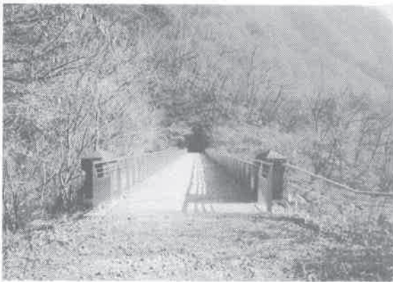
3 rd Usui Viaduct finished deck © Dr Onoda
