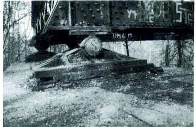
(2) Bilston Glen Viaduct – Old rocker/roller bearing in-situ © Geoff Mather
