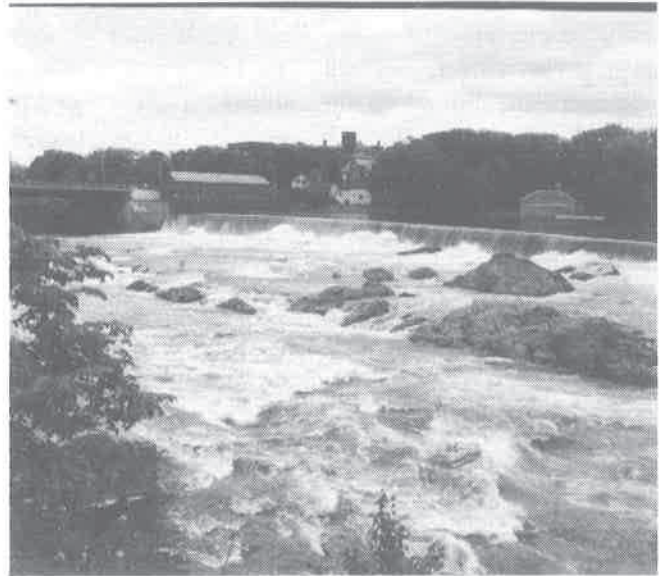
Pawtucket Falls dam and 1848 brick gatehouse at end containing ten 6½ ton sluice gates © Author
