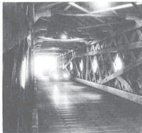
West Cornwall Bridge, CT, USA © Author
