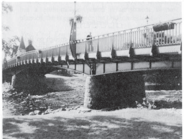
Dalingross Bridge, Comrie after refurbishment in 2001 © The Author
