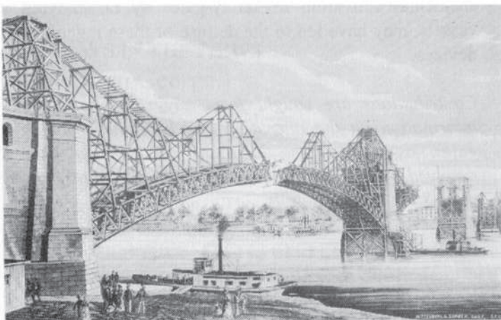
Closing the east arch of the St Louis Bridge. Scientific American , 15 November 1873 © Linda Hall Library
