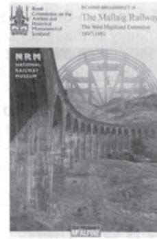
RCAHMS Mallaig Railway Broadsheet – Glenfinnan Viaduct with the timber centering used to build it © RCAHMS [ISBN 1902419316]*
