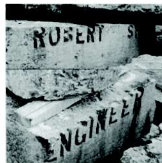
The monumental remains to Robert Stephenson from Britannia Bridge portal after the 1970s fire © James Sutherland
