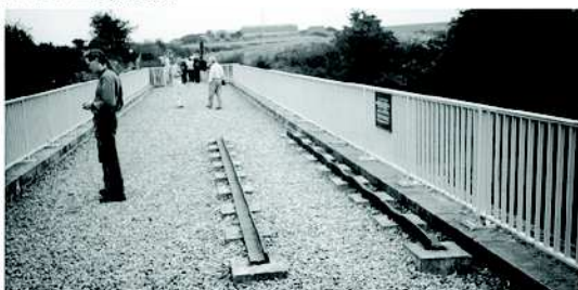
John Ruddy inspecting Laih Milton Viaduct
