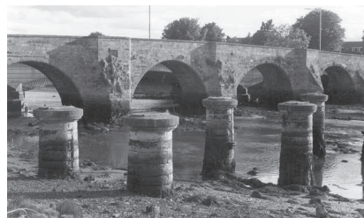
Guard Bridge and St Andrews' railway line © Author
