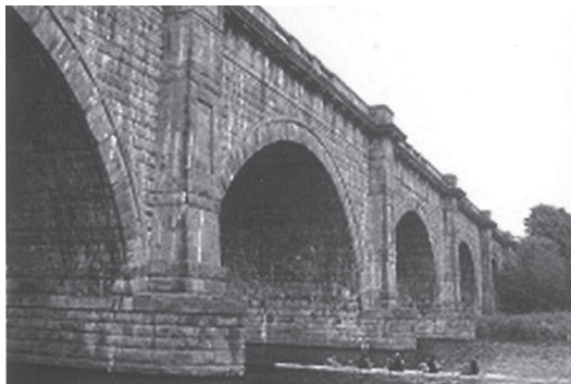
Lune Aqueduct, Lancaster Canal © Paul Dunkerley
