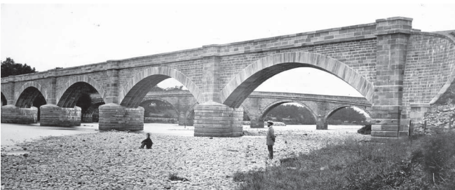
Conon Viaduct & Telford’s bridge (1809–c.1970) © Whyte
