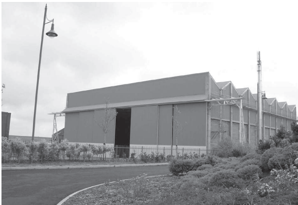
Pembroke Dock Hangar
