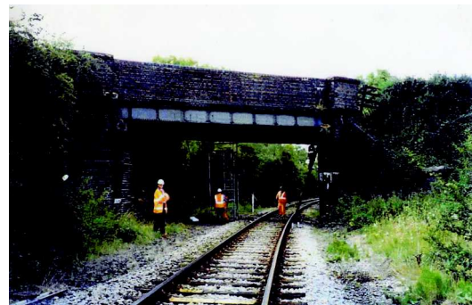
Fritwell Railway Bridge assessment
