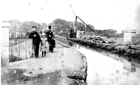
Blackhall Aqueduct Paisley © R Paxton
