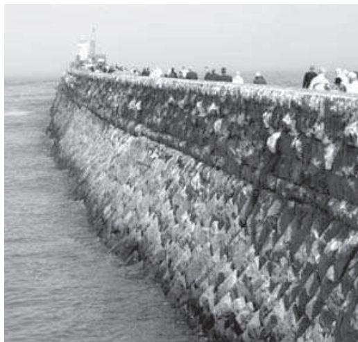
Aberdeen Harbour North Pier – Telford's inclined courses © FM Jones
