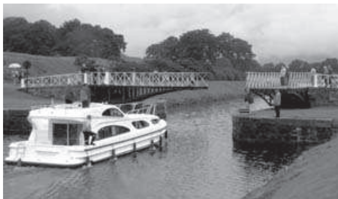
Moy cast-iron turn-bridge, 1820 © FM Jones
