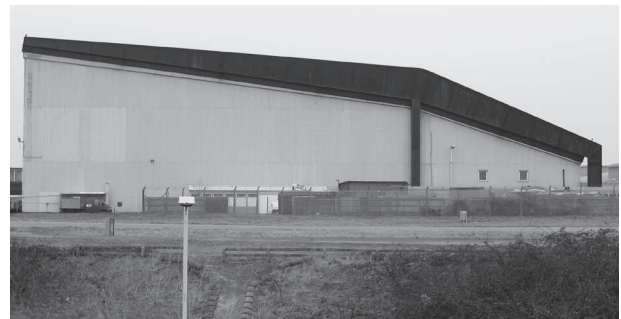
Luton Hangar 89: side view, 14 March 2006
