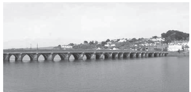
Bideford Long Bridge refurbishment, Devon
