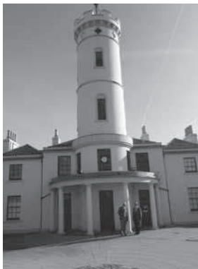
The Signal Tower Museum, Arbroath. Completed in 1813 as the Bell Rock Lighthouse Shore Station © Roland Paxton
