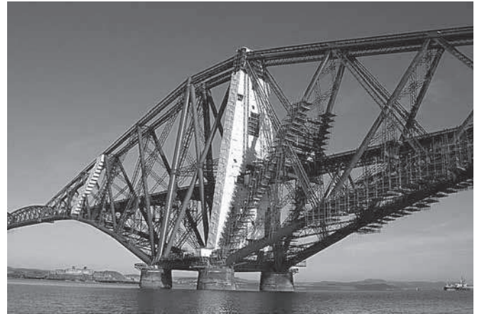
Forth Bridge Restoration
