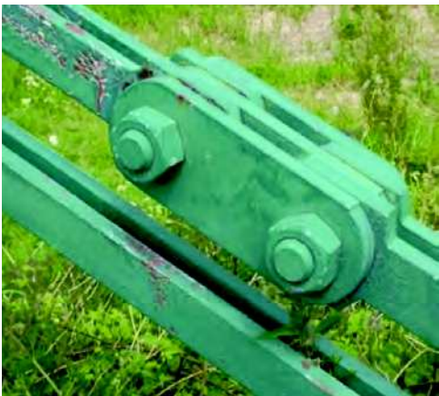
Fig. 3. Twin bar main chains, drilled eyes and use of hexagonal nuts © Redmore
