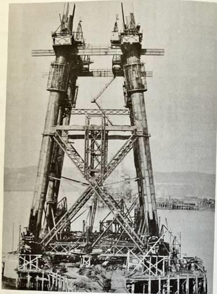
Fig. 14—Queensferry columns, looking through the bridge.
