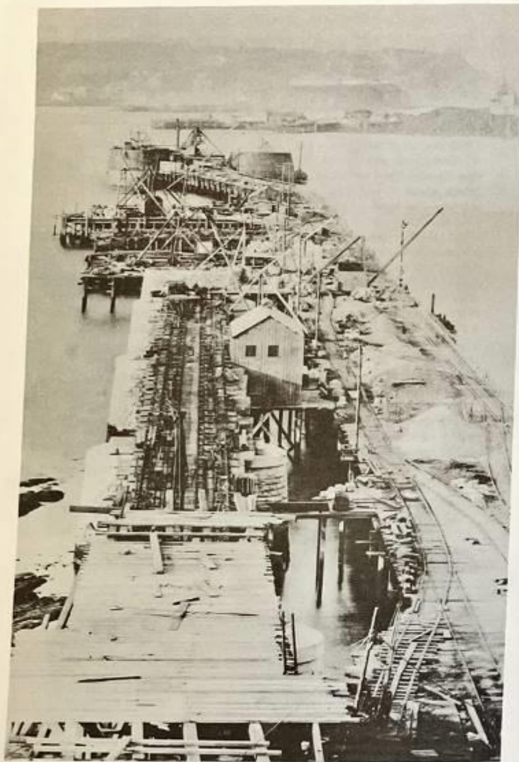
Fig. 11 - View of foundations from South Shore.
