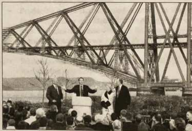
Fig. 2. The Forth Bridge undergoing a £70m refurbishment
