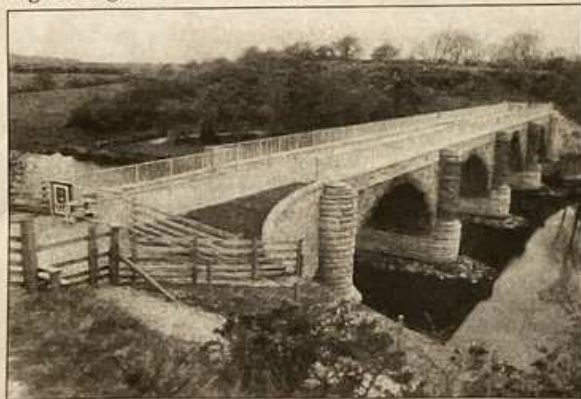
Fig. 6. Laigh Milton Viaduct after conservation in 1996
