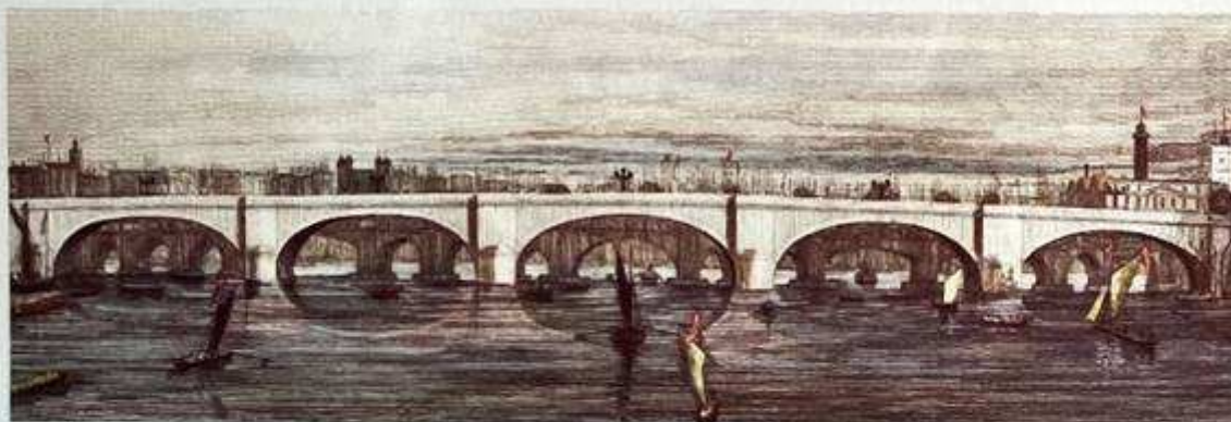
Rennie's magnificent London Bridge, designed in 1820. With centre arch of 152 ft span [ Cresy Ency. 445]. Progressed posthumously to completion in 1831 by his sons. Cost c. £2.5m. Lasted until 1968, when sold and dismantled. By 1971 its facings formed part of a re-build at Havasu City, Arizona. This engraving of 1831 is from a drawing by A. Pugin.
