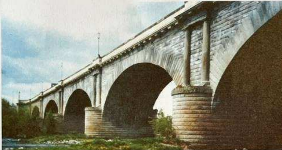
Rennie's first major road bridge at Kelso. Designed in 1798, built 1802-05 with five elliptical spans of 72 ft. Similar in elevation to his Waterloo Bridge, London 1811-17 with nine main spans of 120 ft.
