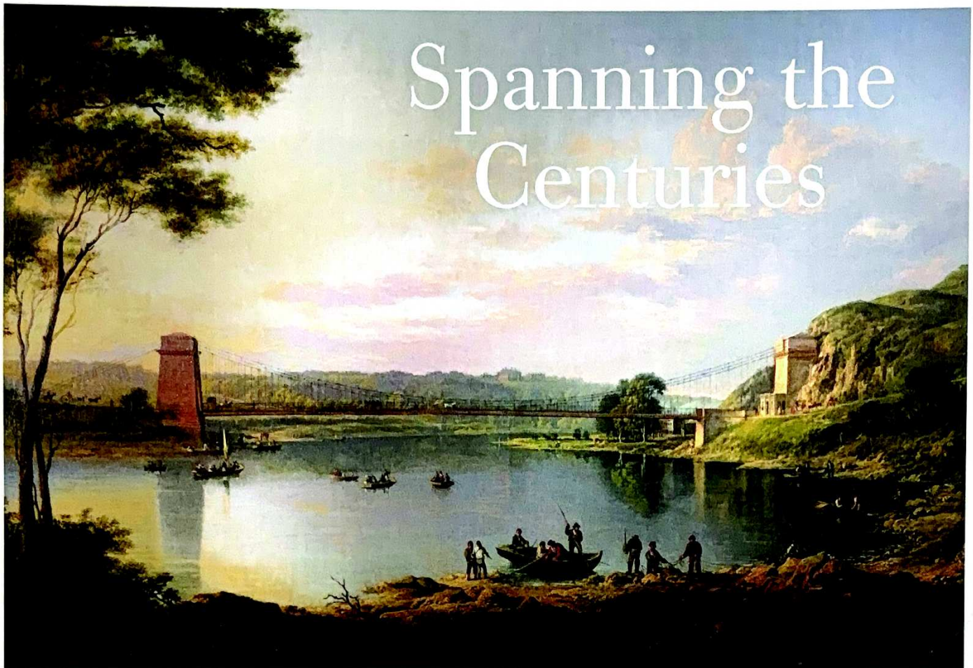
'Union Chain Bridge over the River Tweed' by Alexander Nasmyth (1758-1840). Courtesy The Paxton Trust
