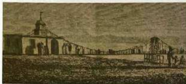
View of 'Land pier' tower building and first 209ft (64m) span; from Capt Brown's specification enrolled in the Court of Chancery, Edinburgh: [Edin.Phil.J VI 1821]
