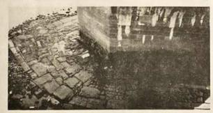
PERTH BRIDGE - Rubble stone sterling protecting a pier base. The stone was packed within the timber cofferdam used to keep out water during construction below water level.
