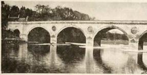
COLDSTREAM BRIDGE 1762-7. Smeaton's first major bridge construction. The base of the left-hand pier, supporting two arches, was built below water level in an open-topped sunken timber box called a caisson. The bridge, sensitively widened in 1960, now carries almost 2m vehicles per annum.
