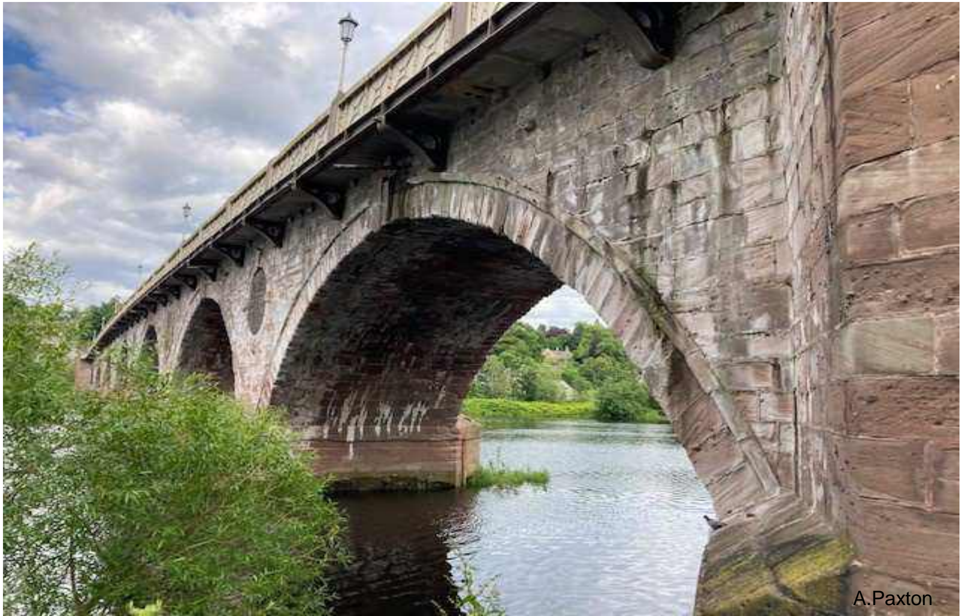
Perth Bridge in 2024 - with Allan Stewart's iron cantilever bracket footways added in 1869
