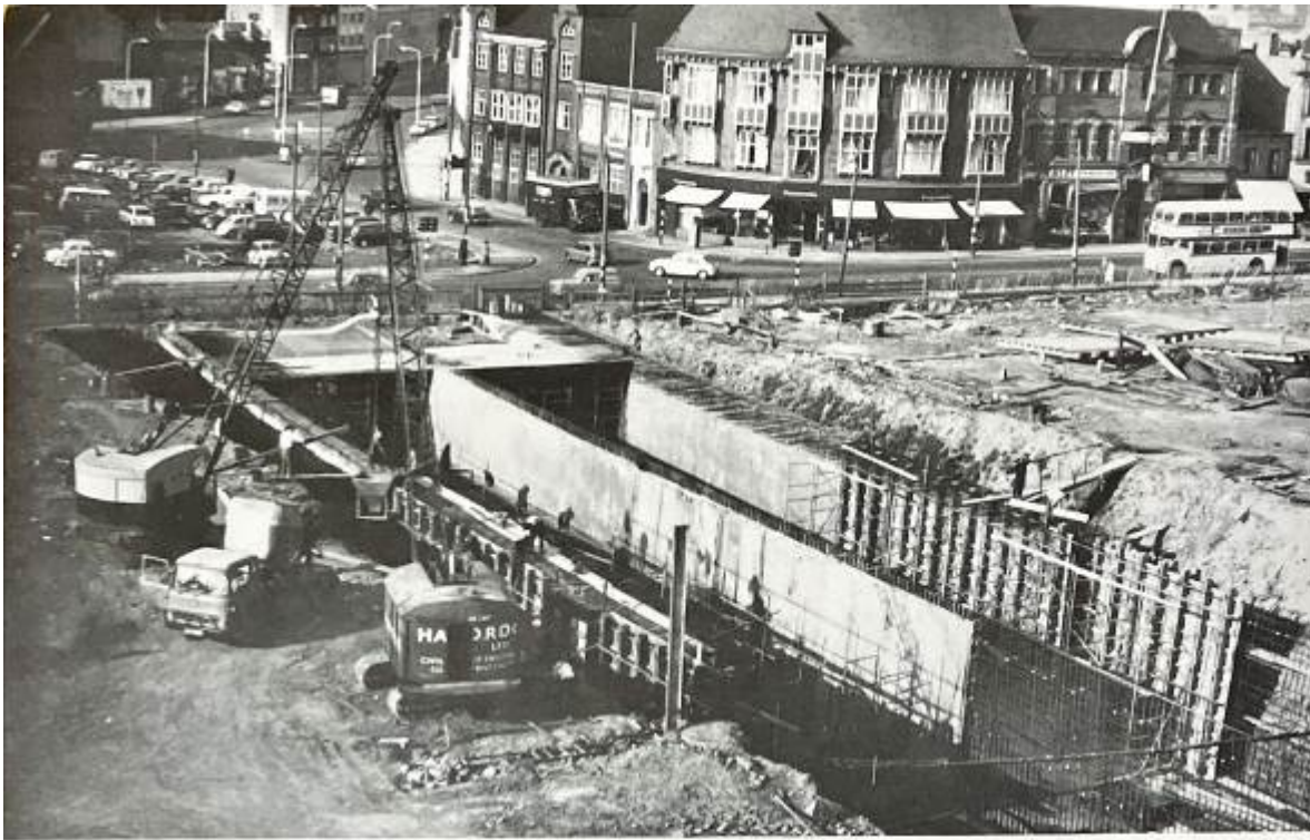
Side walls under construction.
