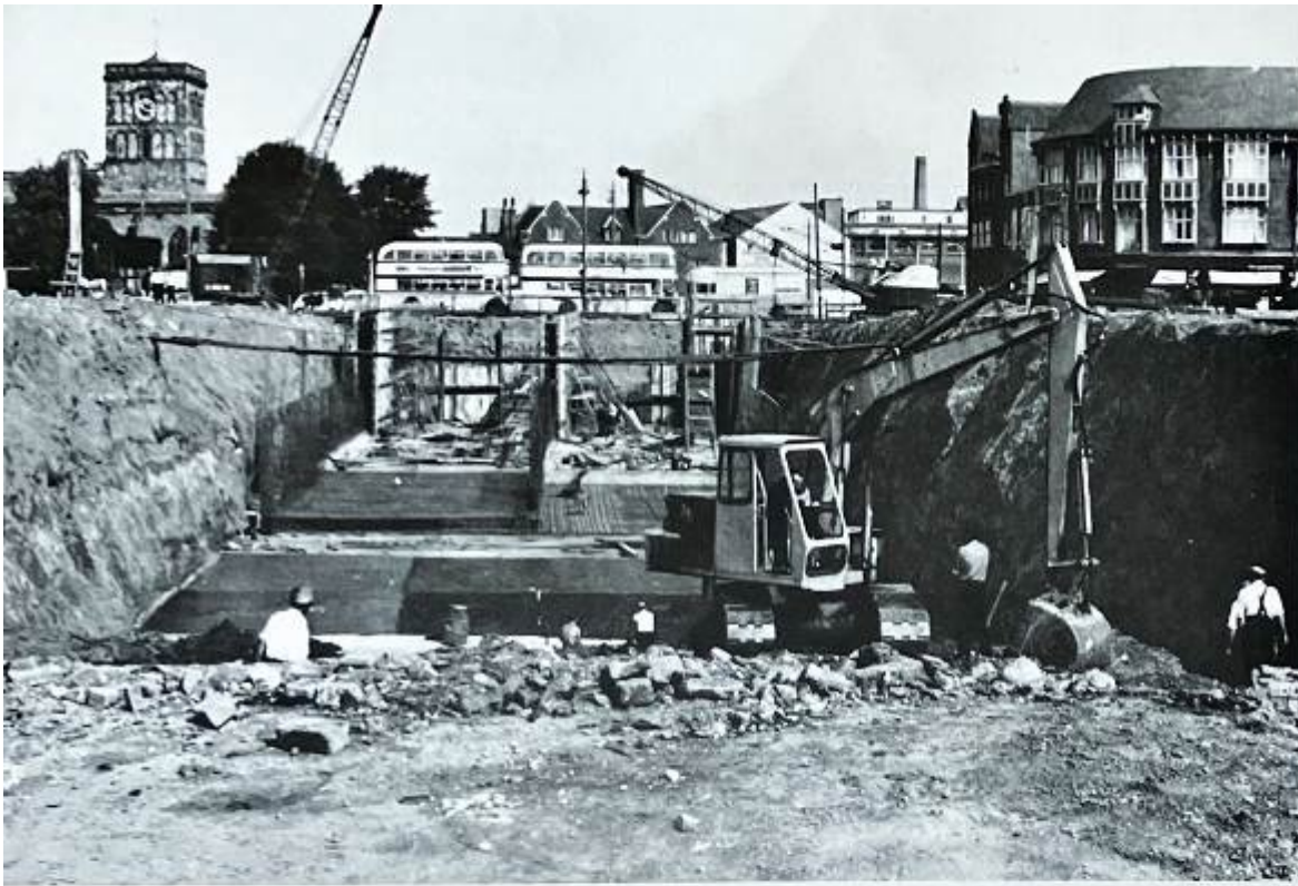
Excavations in progress
