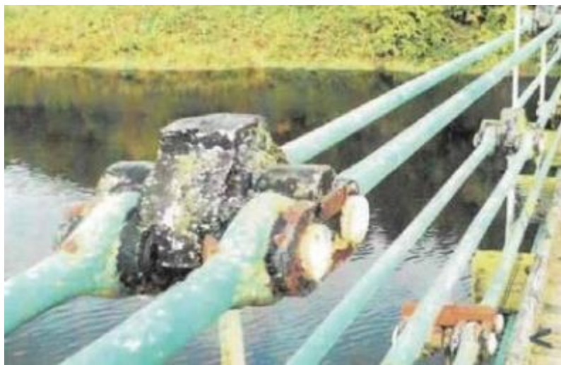
Fig 1 - Union Brodge's 15ft long eye-bar links and connection
