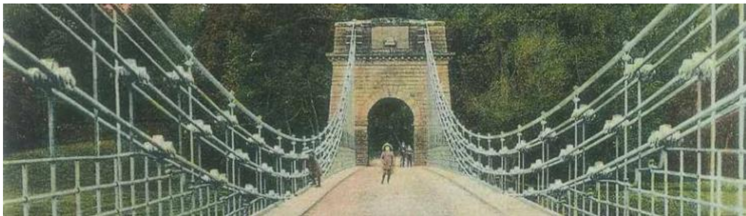
Fig. 11 - The Bridge in 1904 with additional top cables. Capt. Brown's chains at and near mid-span still acted as a safety barrier, obviating the need for their part obscuration by railings. The 1820 deck at mid-span was 1¼ ft lower than shown here [Fig. 5]. Today's deck is 1 ft higher than shown here and, unless the 1820 or 1904 levels are reverted to, railings will be needed after removal of the cables. Note the original deck hangers incorporated into the railings which, with hindsight a poor design concept, now usefully exemplify 1820s practice.
