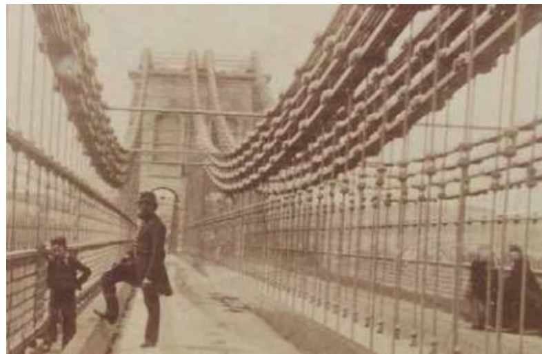
Fig 2 - Menai Bridge's 16 chains each of 5 cross-bolted links
