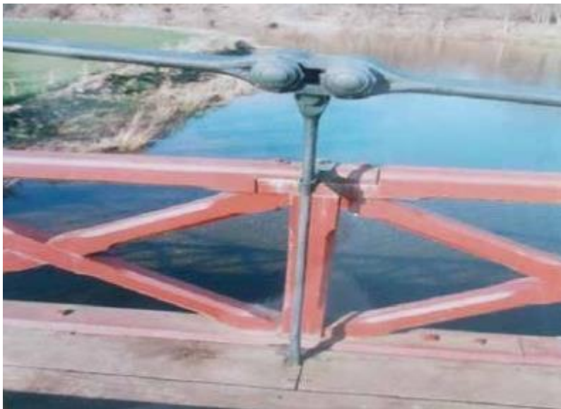
Fig 4 - Kalemouth Bridge (c. 1830 - chains cross-bolted, timber trusses)
