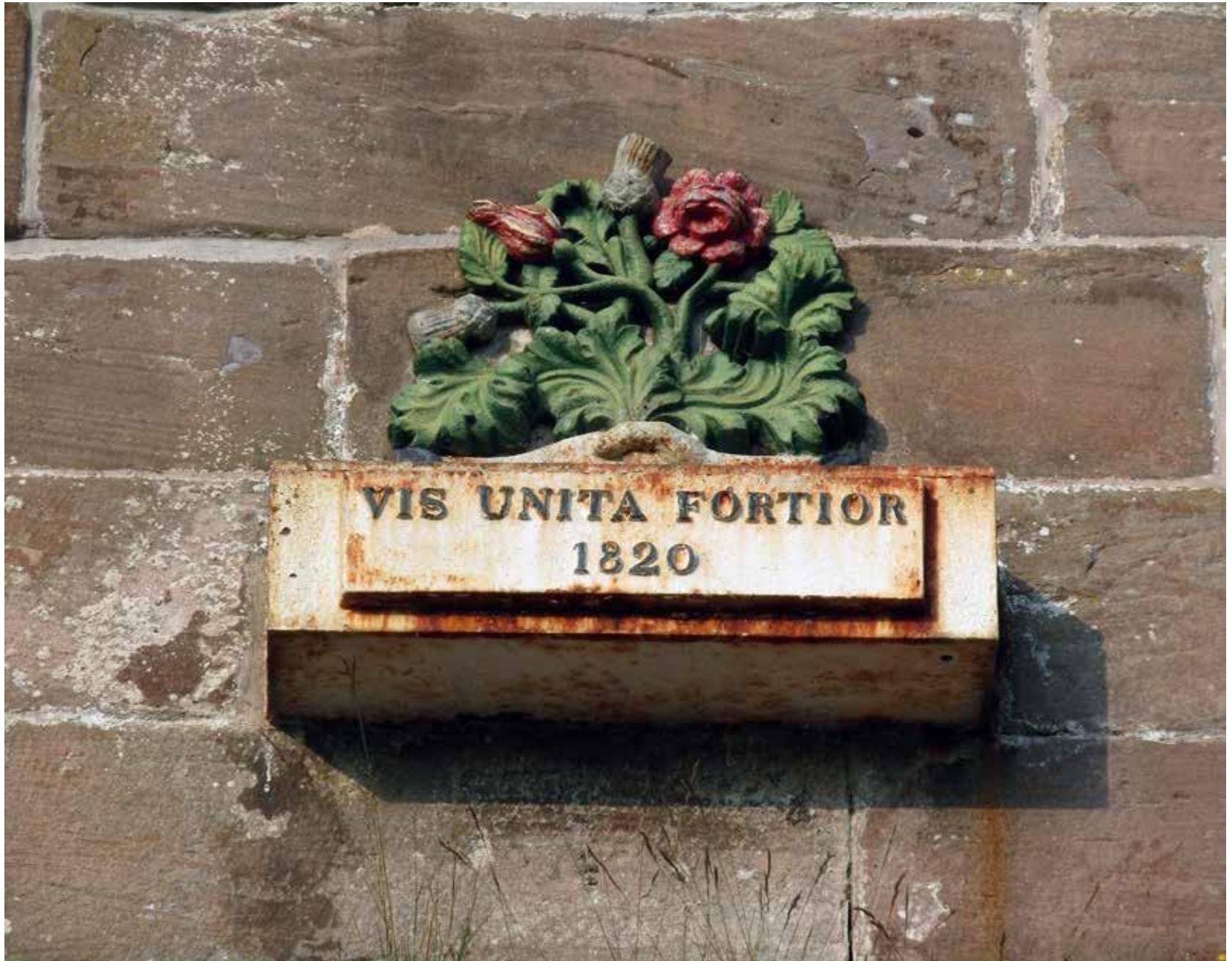
The cast iron plaques bearing the inscription "Vis Unita Fortior" ("United Strength is Stronger") were removed from the railings in the centre of the Bridge (see page 13) at an unknown date (but possibly 1871) and placed in their present locations high on the English and Scottish towers
