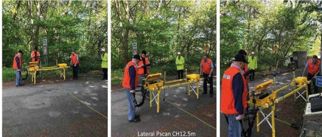
Fig. 2 [L] Start of moving lateral Scan at 12.5m [M] Mid-road scan position [R] End of scan at upstream chain plate intersection position
