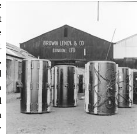
Brown's established his first purpose built chainworks at Millwall on the on the Isle of Dogs alongside the Thames. Here Brown's experimental chain suspension bridge span was erected and tested. Millwall was still manufacturing maritime related products such as buoys when this photograph was taken in 1977, the works closing in the early 1980s. (SKJ photograph)
