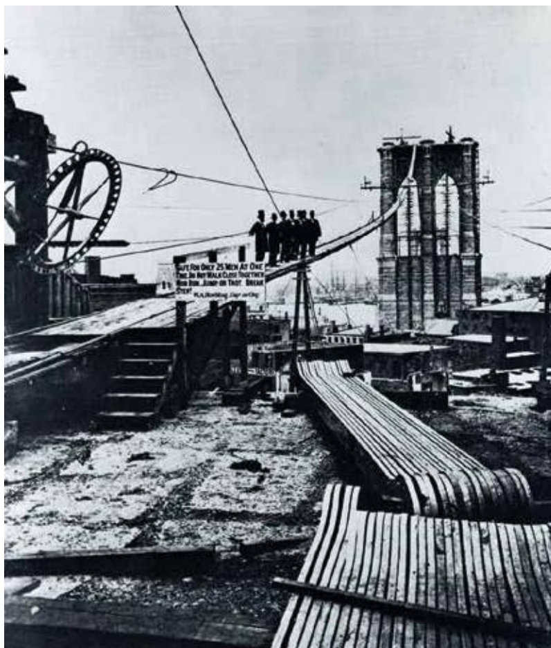
By early 1877 the foot bridges were installed to allow access to install the bridge cables. The wire spinning wheel is shown on the left. In the lower right, wrought iron eye bars are being stored for placement in the cable splay chamber.
