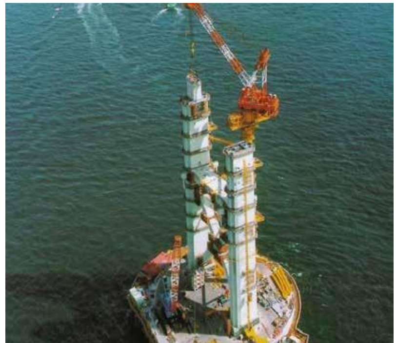
Construction of Tower, Steel blocks were "piling up" (Source; JBEC)
