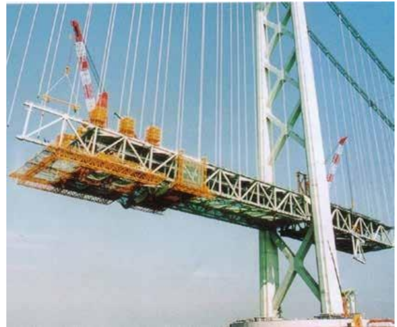
Stiffening Girder Erection Truss advancing outwards from tower (Source: JBEC)
