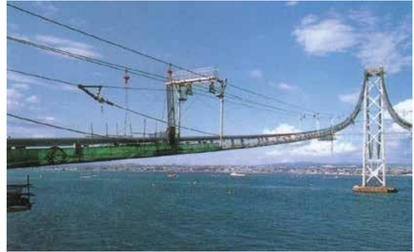
Cable Erection, Spinning wires/strands (Source: JBEC)
