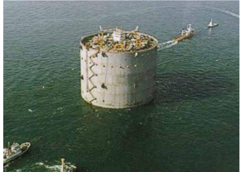
Steel Caisson in floating, Towing 80m diameter "tub" (Source; JBEC)
