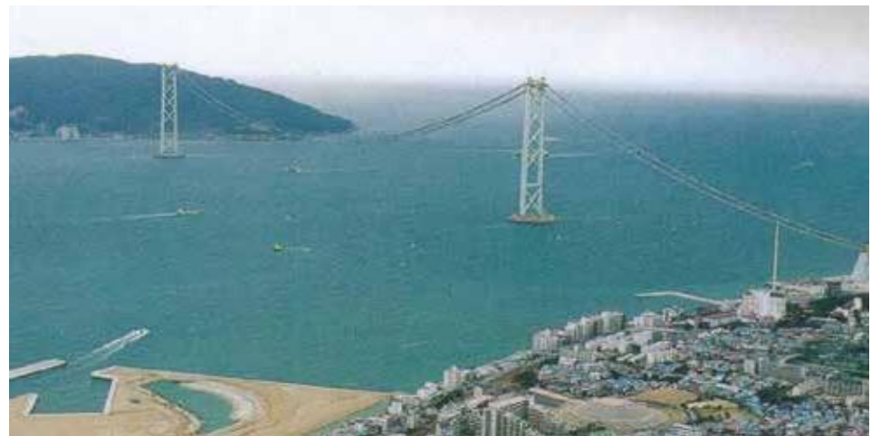
Left: Earthquake disaster in Kobe city (source; JSCE)
