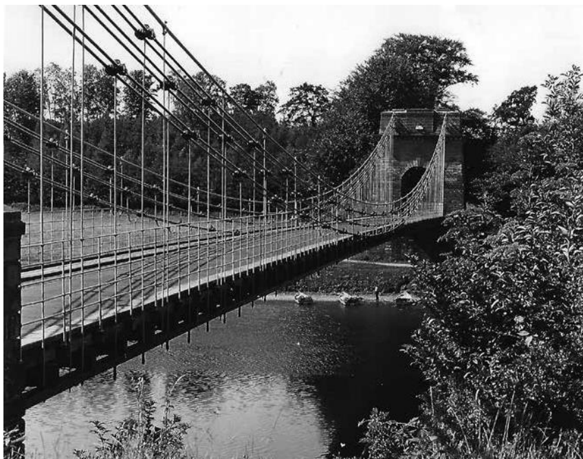
Union Bridge 1974; salmon boats moored below. Salmon netting, which was first recorded at Scotch New Water in 1250, ceased in 1987 (© John R Hume)
