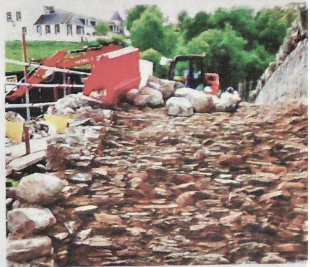
Fig. 9 Tordarroch Bridge repair in 2022 after a parapet collapse – Note the traditional, undressed, arch ring top of tightly packed thin stones under the roadway after c.240 years in service ©The Highland Council
