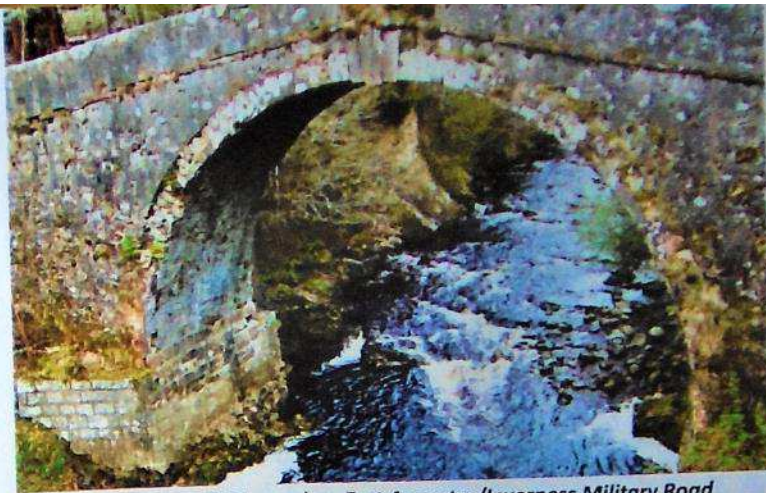
Fig. 2 White Bridge (40ft span) on Fort Augustus/Inverness Military Road ©Sandra Purves
