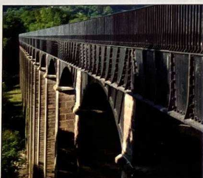
Fig. 1. Pontcysyllte remains Britain's longest and highest aqueduct—the 307 m long, 38 m high cast-iron and masonry structure carries the Llangollen (formerly Ellesmere) Canal over the Dee valley in Wales
