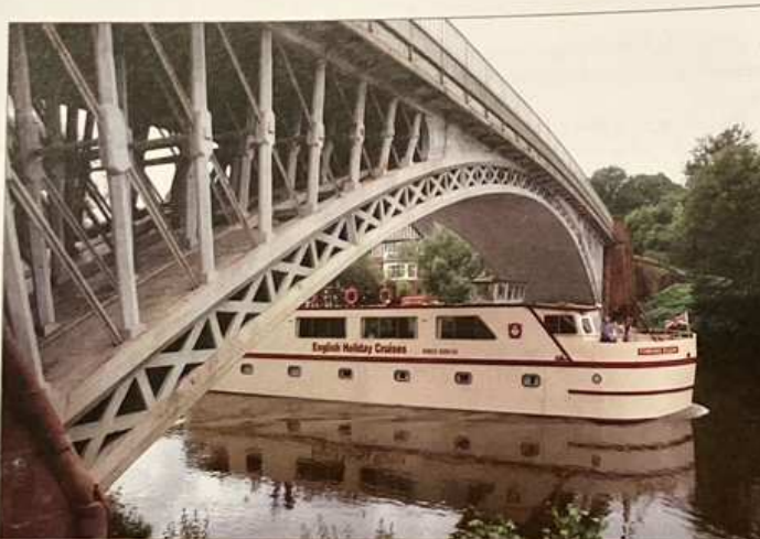
Fig. 11. Holt Fleet Bridge (1829) has a standard Bonar 46 m span and, with the tops and bottoms of its iron ribs now encased in reinforced concrete, remains open to full road traffic
