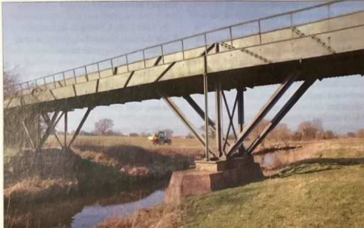
Fig. 2. Longdon-on-Tern Aqueduct on the Shrewsbury Canal was Telford's first cast-iron aqueduct—completed in 1795, it was operational for 170 years and is now a listed ancient monument
