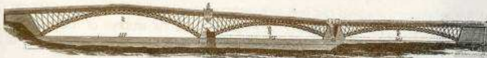
Fig. 2-4 Esk or 'Metal' Bridge (1822-1916) on the Glasgow to Carlisle Road [10 th Report of Commissioners for Repair of Roads and Bridges in Scotland. House of Commons, 25 March 1824]
