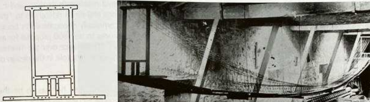
Fig. 3-1 Telford's wire bridge model 1814 preserved at Ellesmere ca. 1906, and cross-section at a support showing 0.1 in (2.5 mm) wire positions [British Waterways Archive, Gloucester Docks, WP 64/53]
