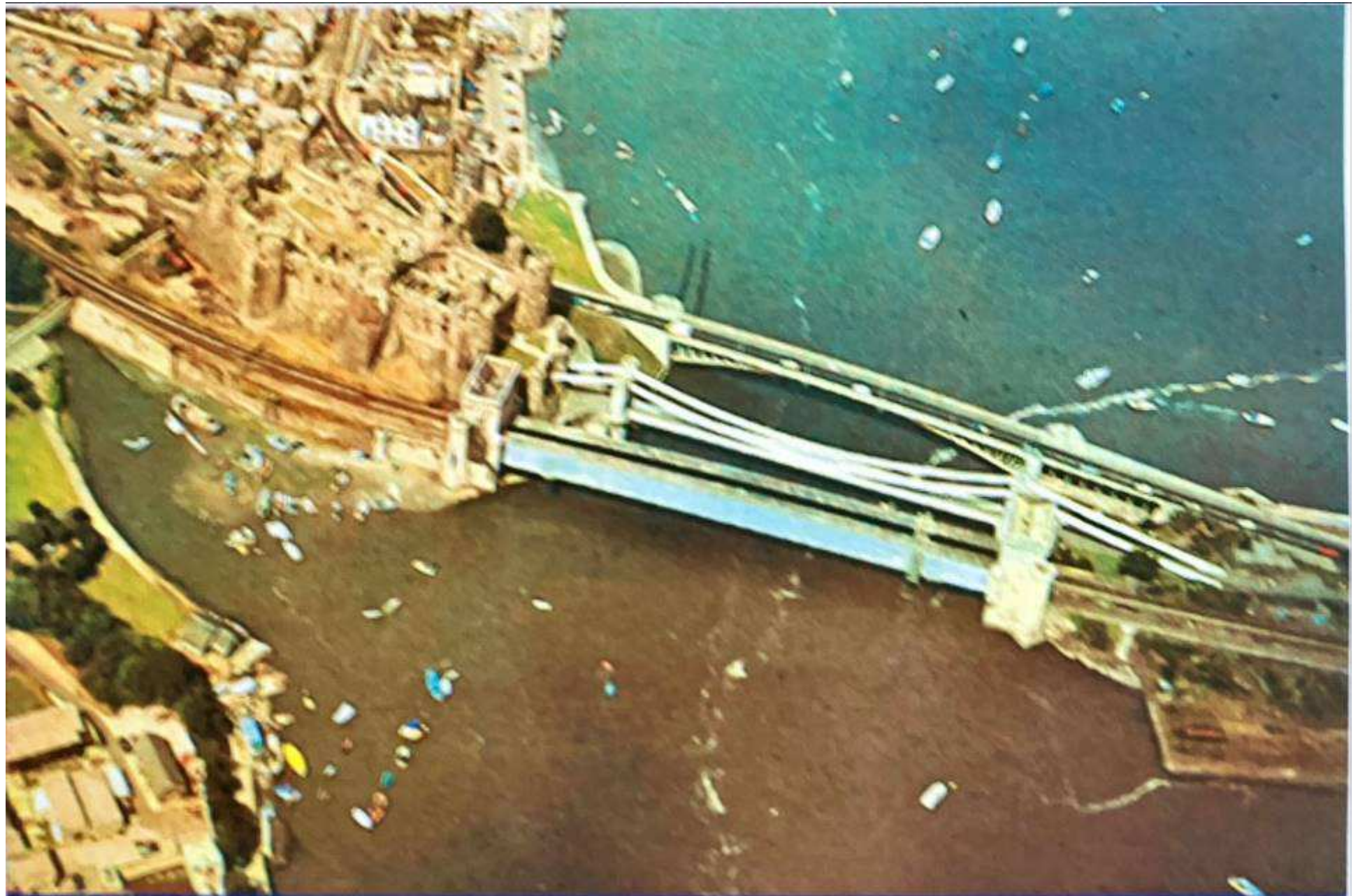
Conwy suspension bridge 1826
