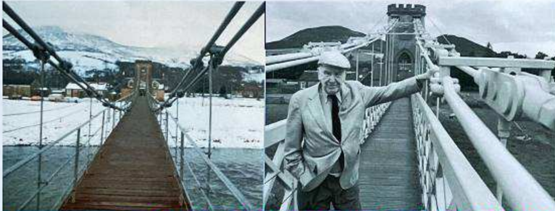
Gattonside Bridge 'before & after' 1990 & 1992 – original ironwork preserved at ICE Museum, Heriot-Watt University
