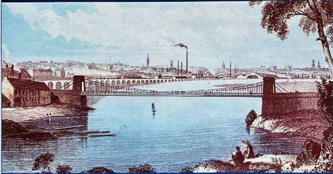
Wellington Suspension Bridge, Aberdeen 1830-1 (Capt. S. Brown). Conserved 2005 by Aberdeen Council
