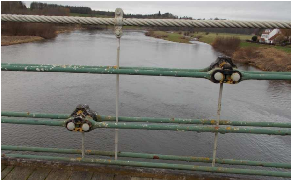
Fig. 8. Union Bridge's 1820 chains with 1903 strengthening cable
