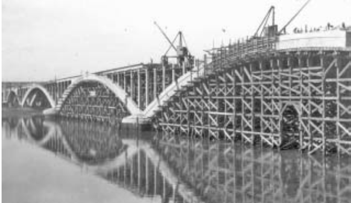
Royal Tweed Bridge under construction
