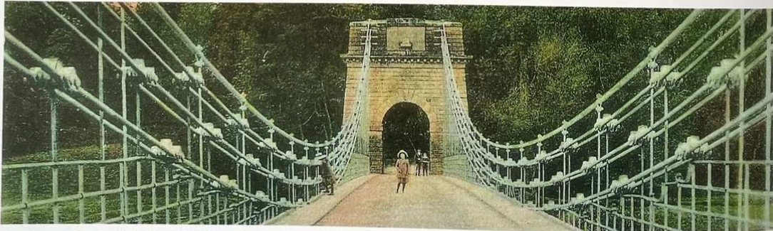
Fig. 11 - The Bridge in 1904 with additional top cables. Capt. Brown's chains at and near mid-span still acted as a safety barrier, obviating the need for their part obscuration by railings. The 1820 deck at mid-span was 1¼ ft lower than shown here [Fig. 5]. Today's deck is 1 ft higher than shown here and, unless the 1820 or 1904 levels are reverted to, railings will be needed after removal of the cables. Note the original deck hangers incorporated into the railings which, with hindsight a poor design concept, now usefully exemplify 1820s practice.
