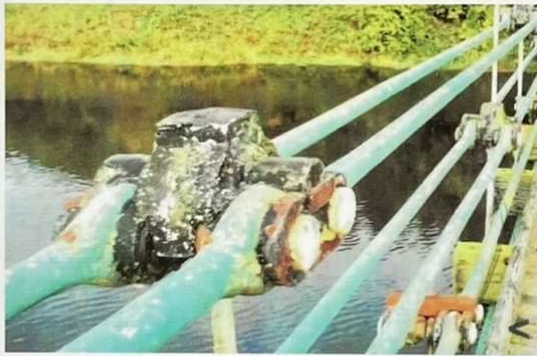
Fig 1 - Union Brodges' 15ft long eye-bar links and connection
