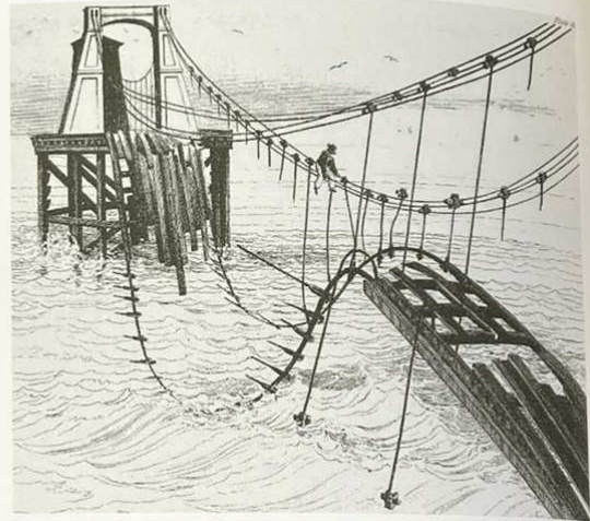
Fig 6 - Brighton Chain Pier (1823-96) - damage in October 1833 [Weale's Bridges 1843]
