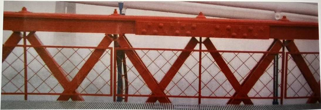
Fig. 7 - Wheeling Bridge WV USA 1849 1010ft span - Upper part of longitudinal Howe type timber trussing (rehabilitated) seen by the author in 1999. Note the adoption of wrapped, parallel multi-iron wire, main cables.
