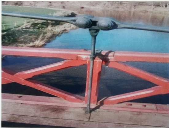
Fig 4 - Kalemouth Bridge (c. 1830 - chains cross-bolted, timber trusses)
