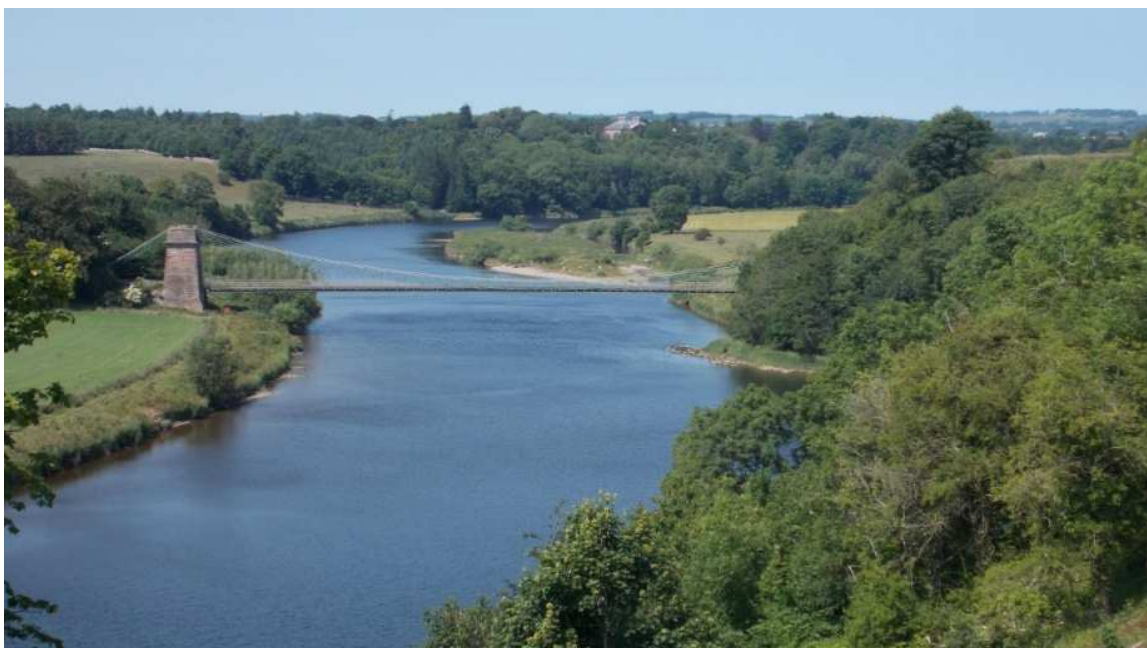
Fig. 9. Union Bridge in 2015
