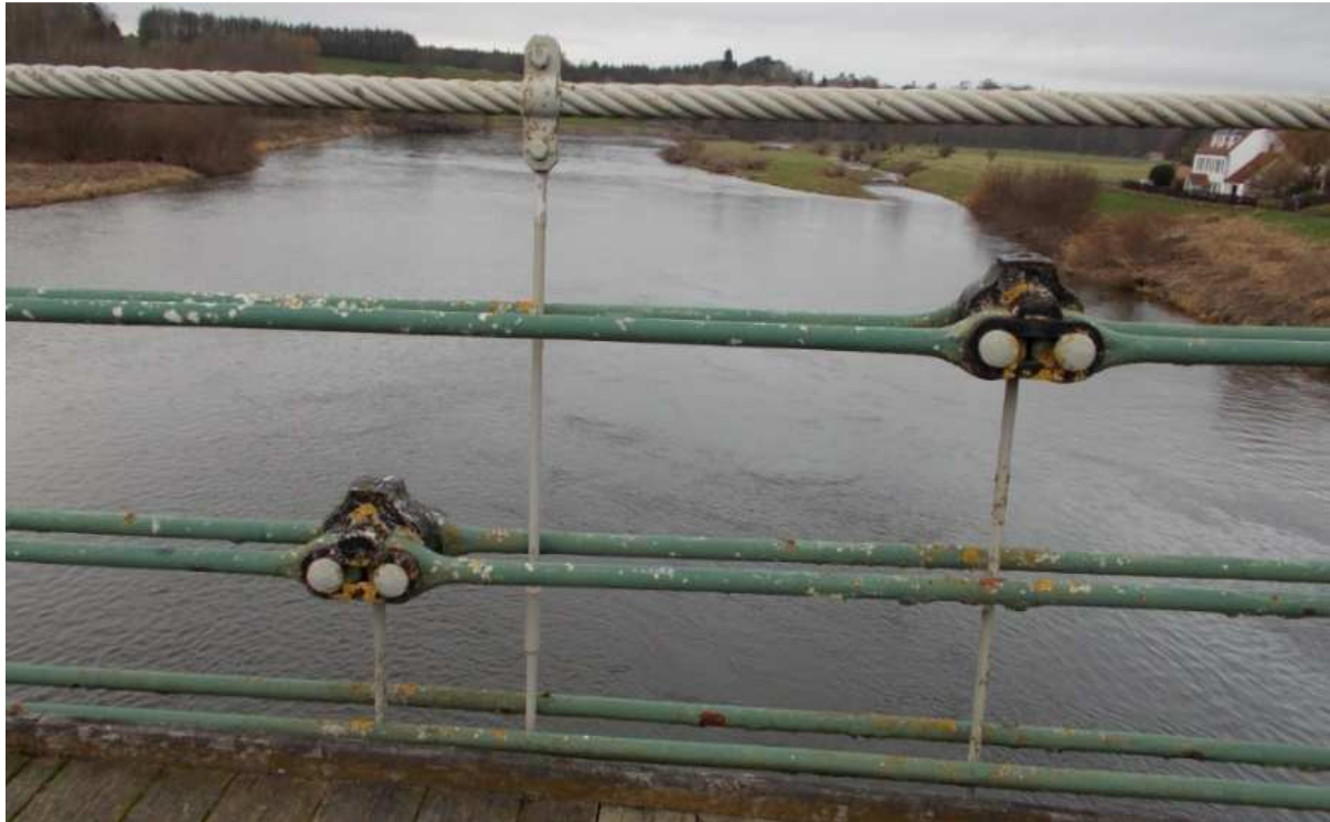
Fig. 8. Union Bridge's 1820 chains with 1903 strengthening cable
