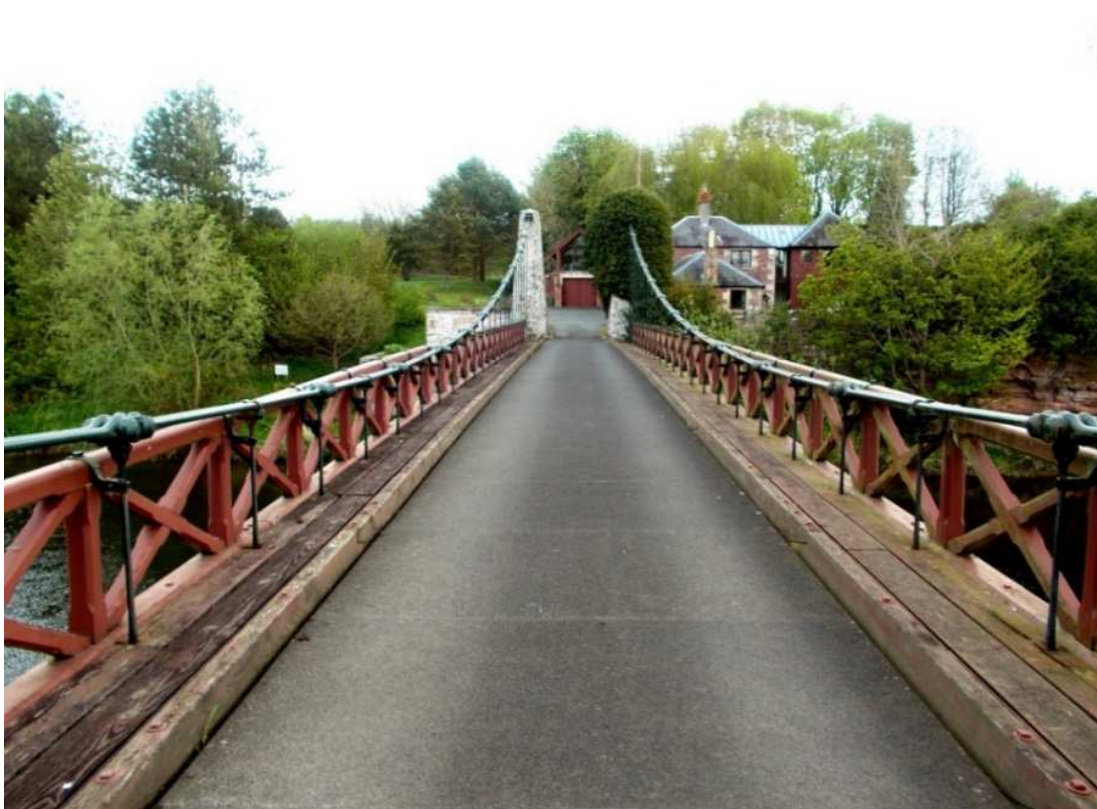
Fig. 4. Kalemouth Bridge in 2016
