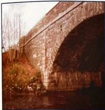
Cay's Glenlair road bridge – 45ft span © K. McCrae
